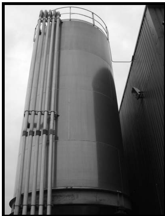
Figure 4.14 Hopper containing granules Courtesy of Kingspan Environmental
