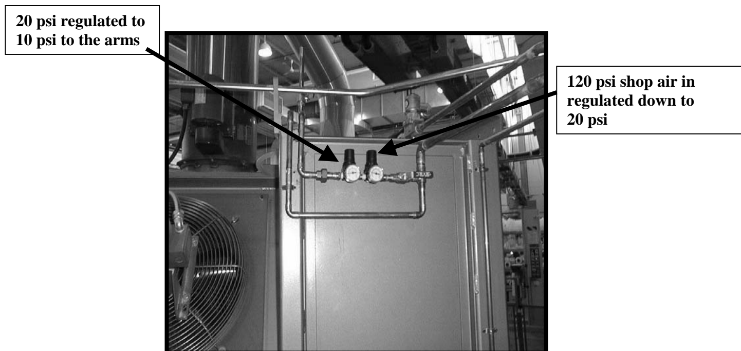
Figure 3.33 Pressure regulators reduce factory air pressure from 120 psi to 10 psi Courtesy of NOVA Chemicals
